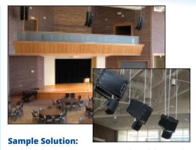
In a large church multipurpose room, the only location for the FOH mixer was on a mezzanine level that did not receive any direct coverage from the main LCR speaker arrays.
